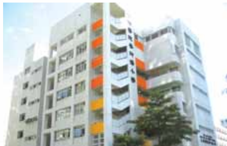
本校新翼外型 The New Wing of Our School
